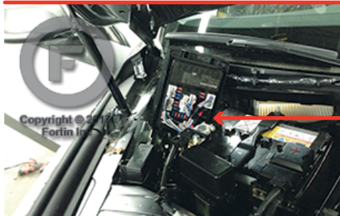
⑦ IPDM-E/R located Engine compartment IPDM-E/R Situé Sous le capot
